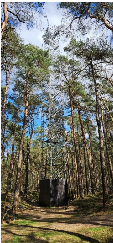
250 Figure 8. The Loobos tower, picture taken towards the East (31 March 2025).
