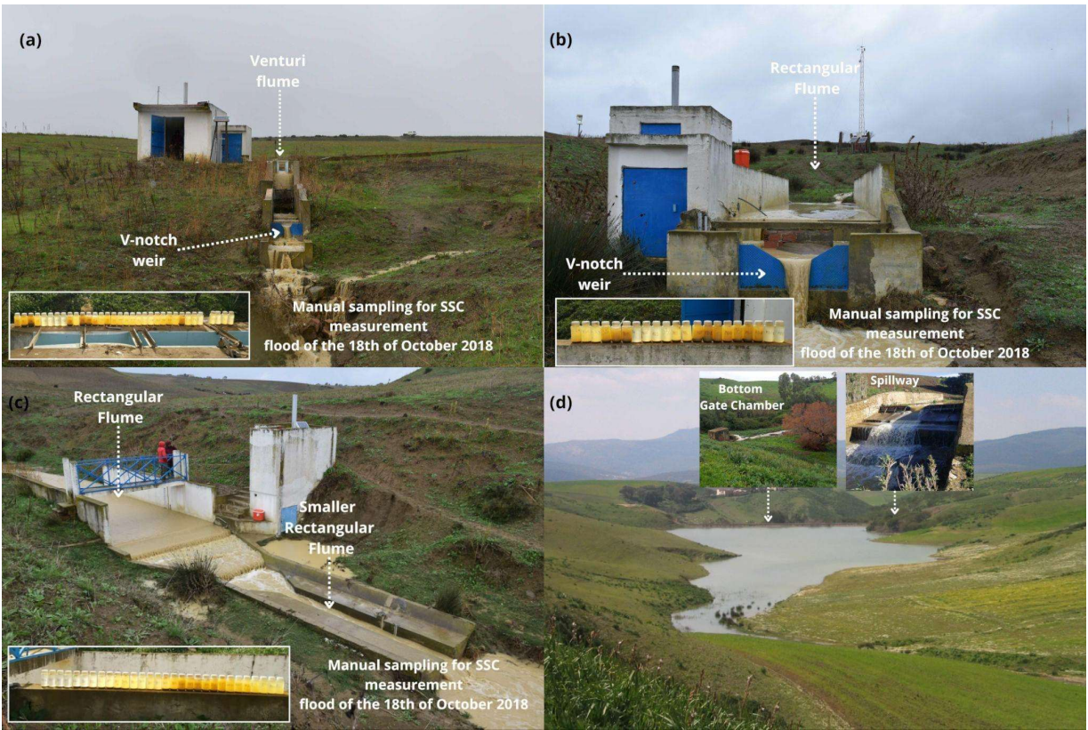
Figure 2. Series of photos illustrating the four hydrometric stations in the Kamech catchment observatory : (a) PAR station, (b) MBV station, (c) GBV station, (d) LAKE station.
