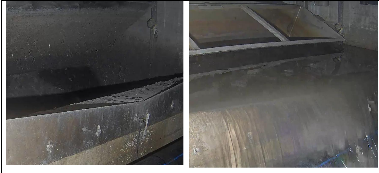
Figure S 23: Left: the Decagon sensor, i.e. Meter 5TM mounted on a weir crest in dry environment; right: submerged sensor in case of an overflow event.
