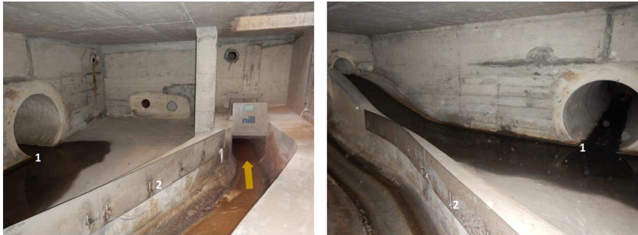
Figure S 17: Overflow chamber RU 40a with slide gates (photos taken from HBT, 2016; modified). The left and right pictures show a downstream and upstream view. The numbers 1 and 2 label same points of reference and the arrow indicates downstream flow direction.
