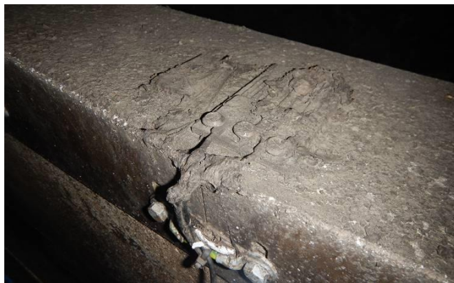
Figure S 47: Left: Capacitive sensor for overflow discharge detection at the weir crest basin RUB 59 after three years of operation. Photo: S. Bloem, Eawag. Right: Cross-section through overflow structure (not drawn to scale), including inflow chamber (2), retention tank (1), overflow to receiving water (3) and US level sensor (h01) and the capacitive sensors (bm332 and dl311).
