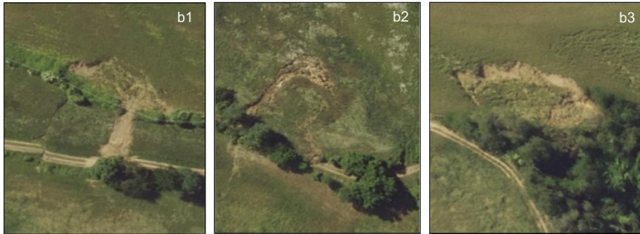
DS2) Debris slides with low-mobility causing limited or no vegetation removal
