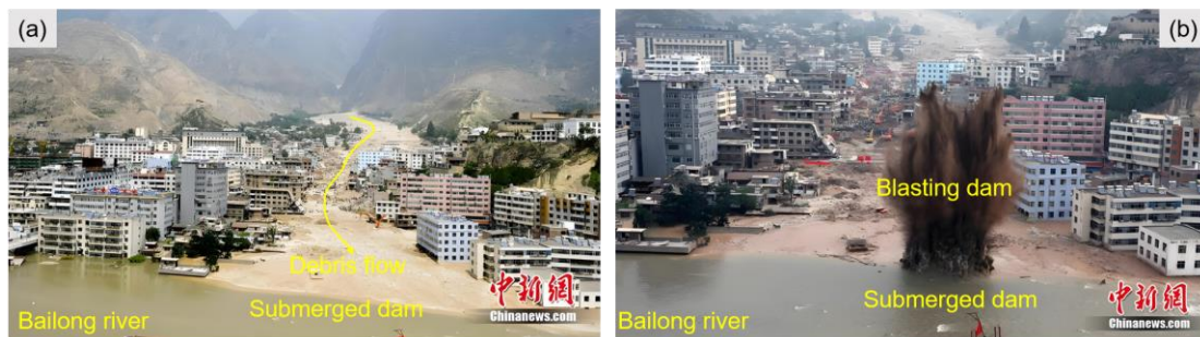
Figure 1. Post-disaster images of the Zhouqu debris flow. (a) The debris flow rushed into the Bailong River, forming a submerged dam; (b) blasting operations on the debris flow barrier dam to accelerate discharge. The images were obtained from China News Service ( https://www.chinanews.com.cn/ ).
