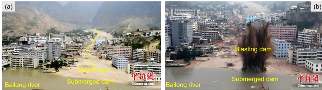
Figure. 1 Post-disaster images of the Zhouqu debris flow. (a) The debris flow rushed into the Bailong River, forming a submerged dam; (b) Blasting operations on the debris flow barrier dam to accelerate discharge. The images are from China News Service ( https://www.chinanews.com.cn/ ).
