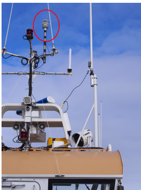
Figure 7. Sensor installed on top of MS Bard, marked with a red circle.
