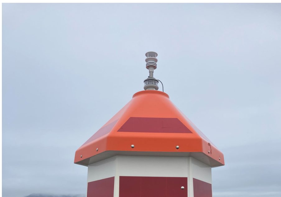
Figure 2. Sensor installed on top of the Gåsøyane lighthouse.
