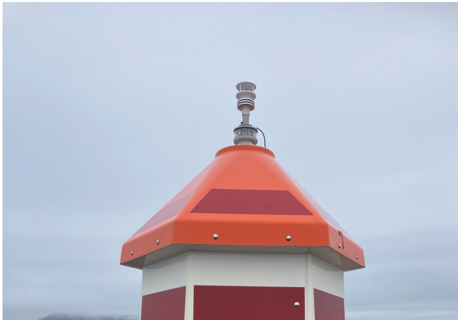
Figure 2. Sensor Weather station installed on top of the Gåsøyane lighthouse.
