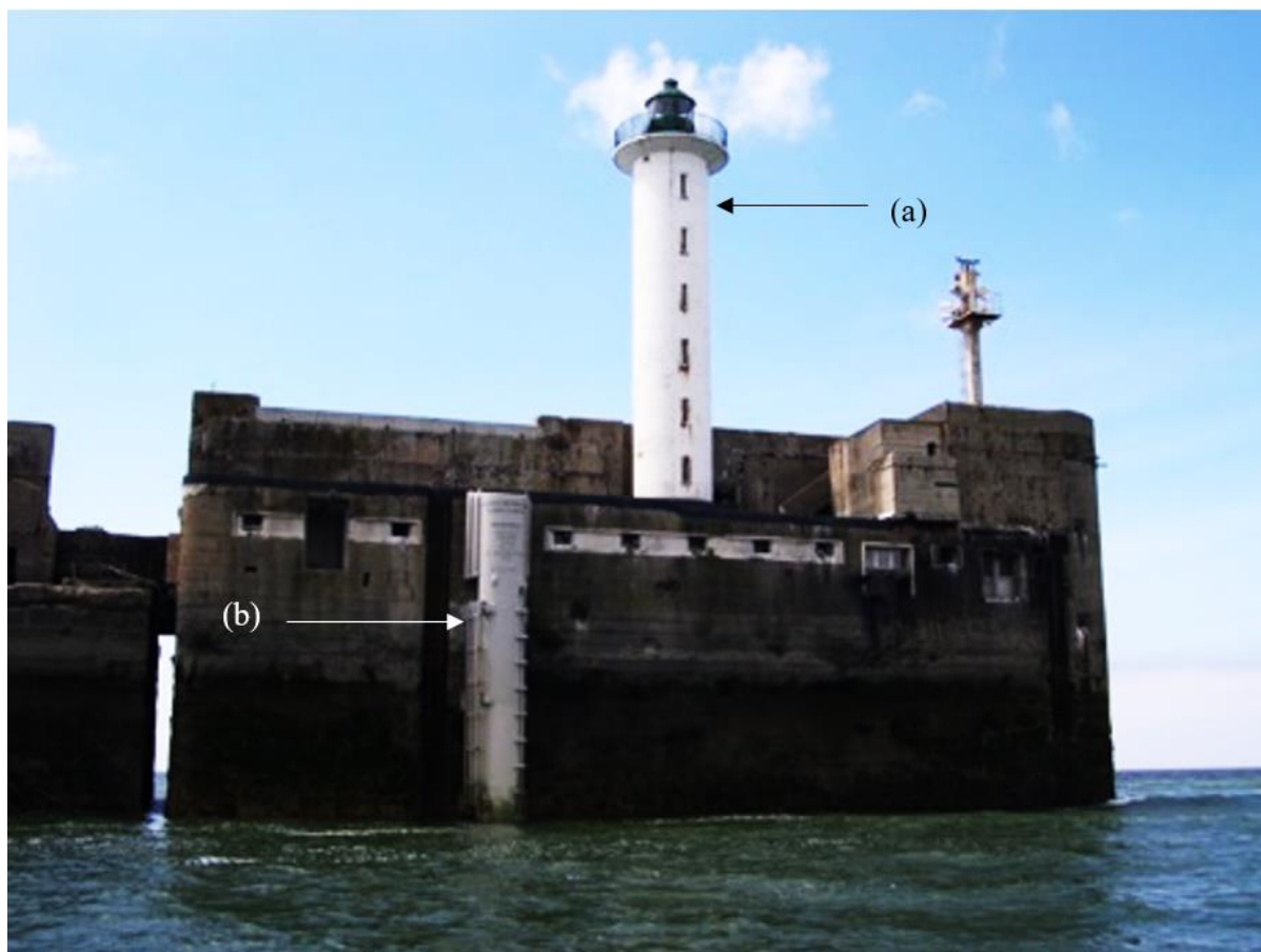
145 Figure 2 MAREL Carnot station consisting of the light house (a), and the MAREL Carnot tube (b) (photo © Ifremer).
