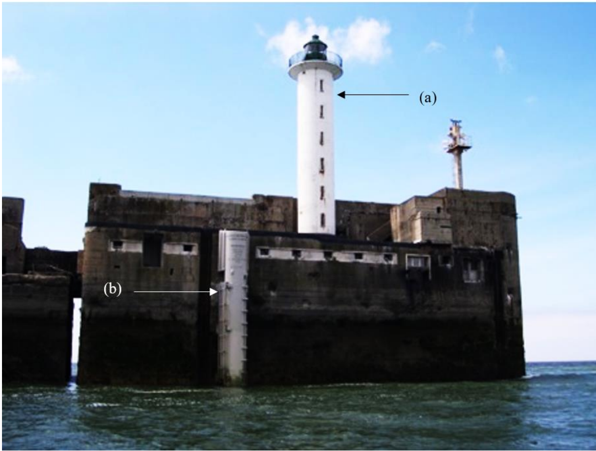
Figure 2 MAREL Carnot station consisting of the lighthouse (a), and the MAREL Carnot tube (b) (photo © Ifremer).
