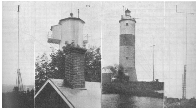
Figure 3. Sandström anemometer installations at four different Swedish stations in 1928. From left to right: Agö (mast), Grimskär (light house), Ölands södra udde (light house) and Lilljungfrun (storm warning mast) (Östman, 1928).
