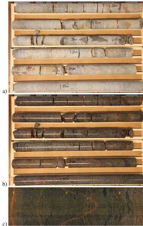
Figure 2. Fracture inspection from drill cores (section from 19 m - 26 m) : a) dry, b) wet. c) Image from borehole televiewer BIPS tool before the experiment in the section where test HF1 was conducted (24 - 26 m) .
