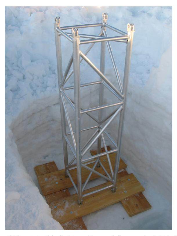
Figure F2. The wooden boards placed at the bottom of the support aluminum tower, at 2 m depth in the firn, during the AWS installation. Photo taken on 30 September 2011.
