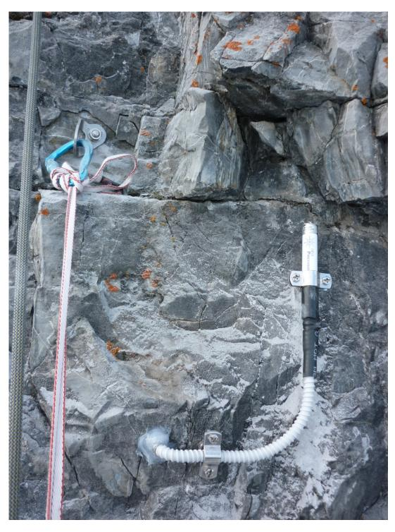
Figure I1. The rock wall temperature datalogger (Geoprecision thermistor string) installed close to the Payer refuge. The datalogger is anchored to the rock wall and is connected to three temperature sensors placed at 0.1, 0.3 and 0.55 m depth inside a horizontal hole drilled in the rock wall. Photo taken on 28 November 2011.
