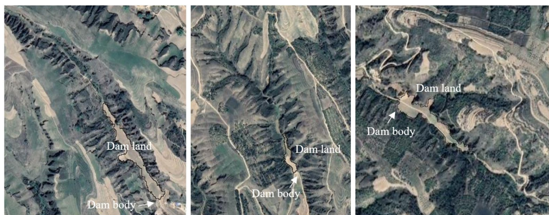
Figure R1: Dam bodies of small check dams.
