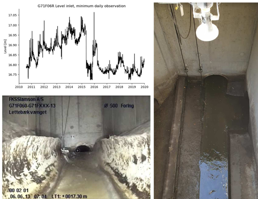
265 Figure 8: Anomaly in level data and possible causes. The minimum daily water level in G71F06R (upper left corner) along with a CCTV image (lower left corner) of G71F06R from June 2013 and a photo of the same location from 2019 (right) showing also the location of the level sensor (radar). Videos and additional photos can be found in the data set (Pedersen et al., 2021a). A large anomaly in data occurs May 11 th , 2015, which is possibly due to retrofitting of the banquettes in the structure at this date. Pictures by (VCS Denmark, 2020)
