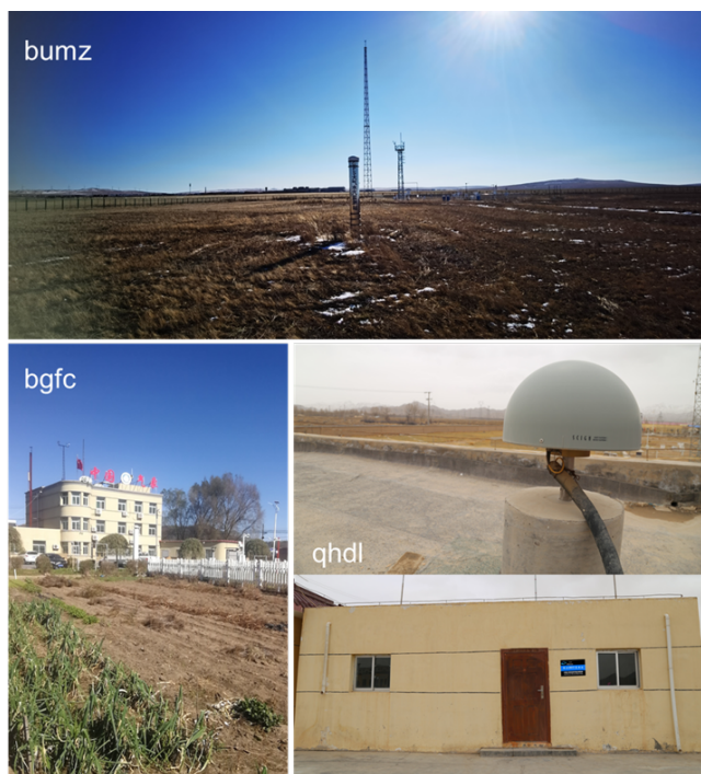
Figure 5. Photos of typical GNSS sites. “bumz” and “bgfc” are two CMA sites, and “qhdl” is a CEA site.
