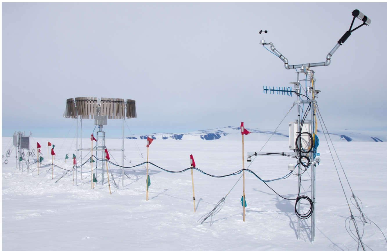
140 Figure 2: A complete APS standard site installation at the Phoenix Airfield site at the completion of the installation in November 2017. The UNAVCO power system is at the far left, the weighing precipitation gauge installed inside the wind shield at the center, and the instrument tower is on the right.
