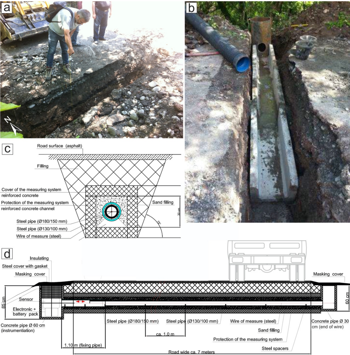
251 252 Figure 5. (a) Opening of trench n. 1. (b) Installation of the concrete protection for the extensometer. 253 (c) Section transversal to the extensometer system. (d) Longitudinal section of the extensometer 254 system. Location of the two measurement stations provided in Figure 3a. 255
