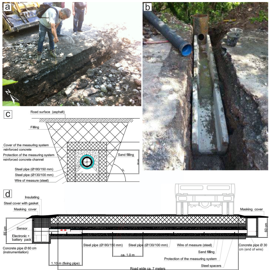
184 Figure 4. (a) Opening of trench n. 1. (b) Installation of the concrete protection for the extensometer. 185 (c) Section transversal to the extensometer system. (d) Longitudinal section of the extensometer 186 system. Location of the two measurement stations provided in Figure 3a.
