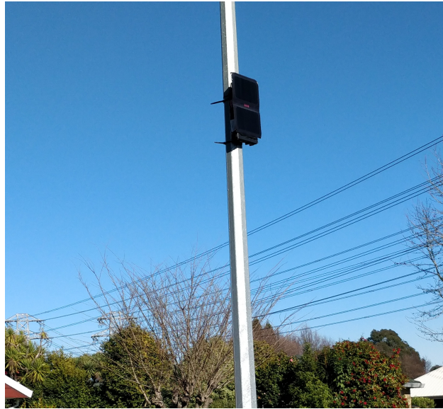
Figure 4. An example of a typical ODIN installation on a light-pole.
