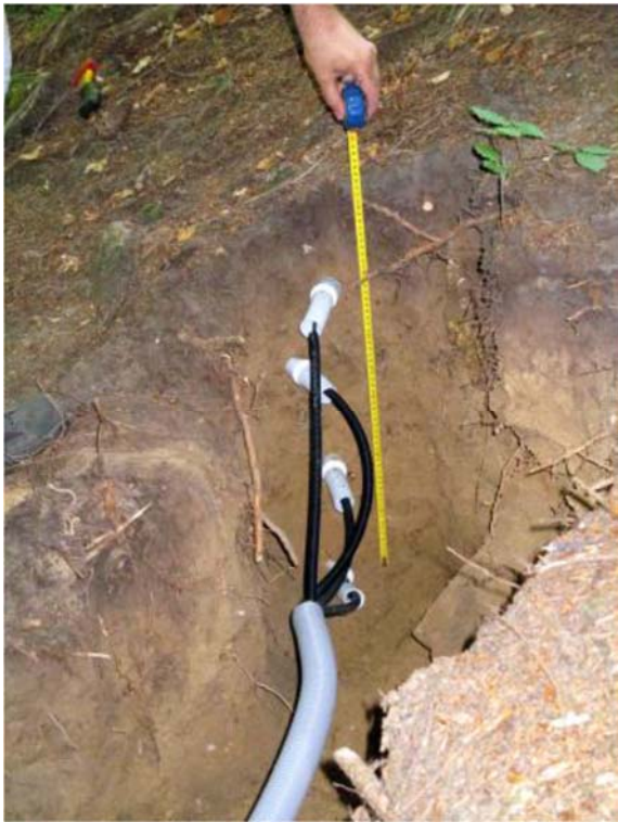
295 Figure 5: HydraProbe sensors installed at site Q2S0
