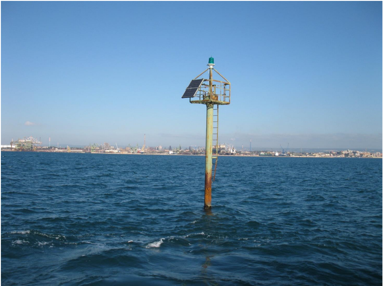
Figure 2: Seamark where the monitoring station in Mar Grande was installed.
