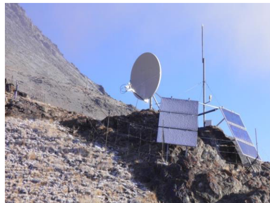
Figure 3: Station type two with a compact weather transmitter connected at the pole between the solar panels at the station Alai-6 (ALA6)
