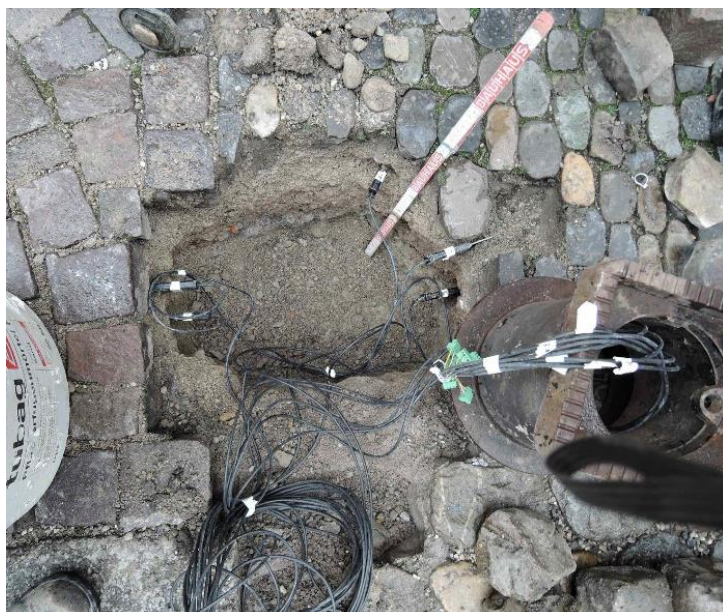
5 Figure 4: Installation of the soil moisture sensors at the plots of cluster D and the small manhole used for accommodating the data logger.
