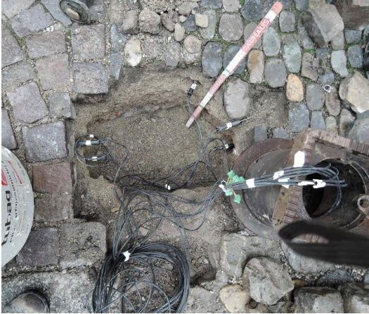
Figure 4: Installation of the soil moisture sensors at the plots of cluster D and the small manhole used for accommodating the data logger.
