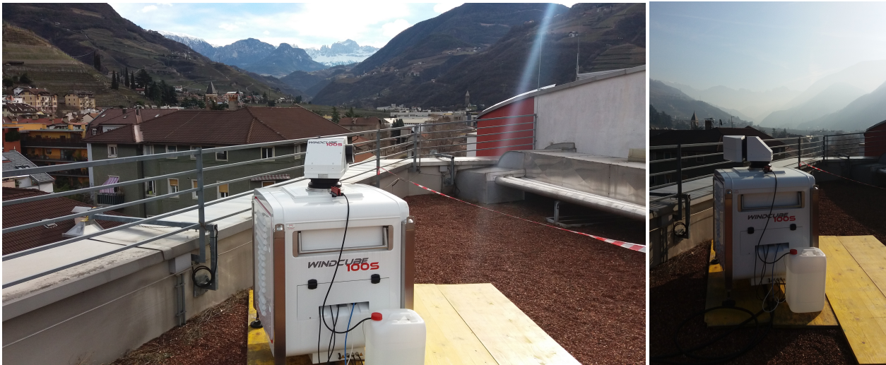
Figure 4. The WINDCUBE 100S Doppler Wind–LIDAR from Leosphere (France) installed on a roof at 18 m AGL. In the background the outlet of the Isarco Valley.
