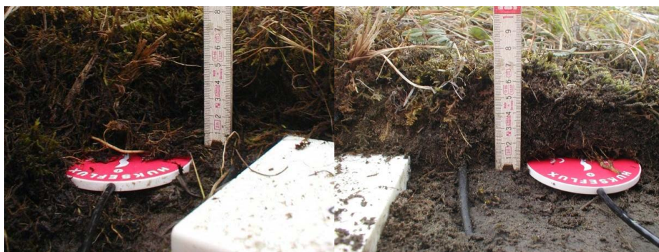
Figure B12. Hukseflux HFP01 ground heat-flux sensors, installed on 24 August 2002.
