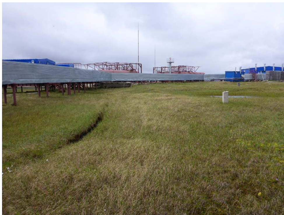
Figure E4. Borehole location (wooden box on right side) with the new Samoylov research station and water supply system (silver metal structure extending above the tundra surface).
