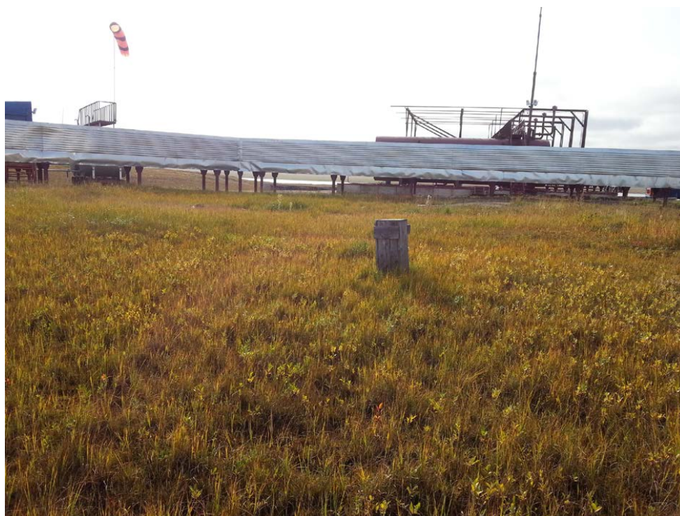
Figure E3. Location of the 2006 borehole (wooden box) showing the proximity of the new 775 water supply system (since 2013: silver metal structure extending above the tundra surface).
