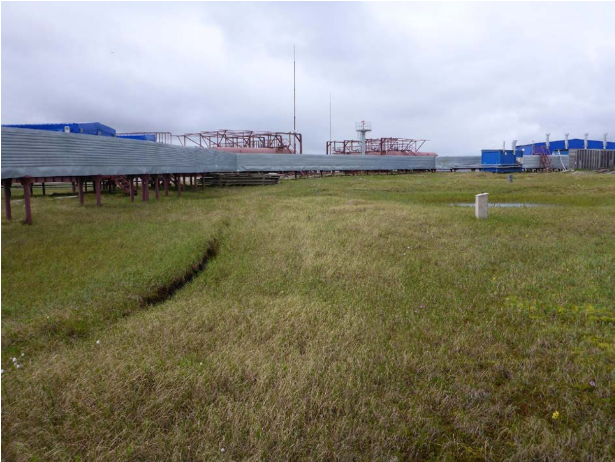
835 Figure E4. Borehole location (wooden box on right side) with the new Samoylov research station and water supply system (silver metal structure extending above the tundra surface).
