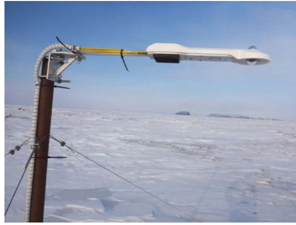
Figure B3. Kipp & Zonen CNR4 radiation sensor (including CNF4 ventilation unit) for measuring incoming and outgoing shortwave and longwave radiation, respectively, installed on 22 August 2014.
