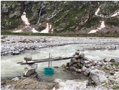
5 Figure 6: The construction of the Djankuat Gauging Station (photo by E.Rets):
