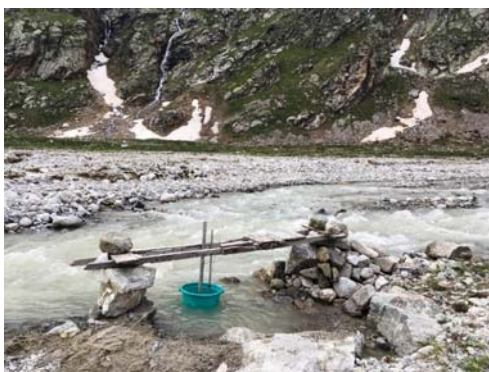
5 Figure 6: The construction of the Djankuat Gauging Station (photo by E.Rets);
