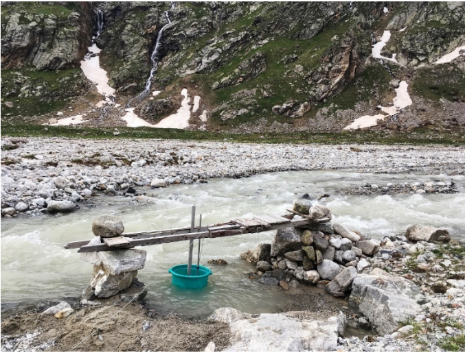
Figure 6: The construction of the Djankuat Gauging Station (photo by E.Rets).
