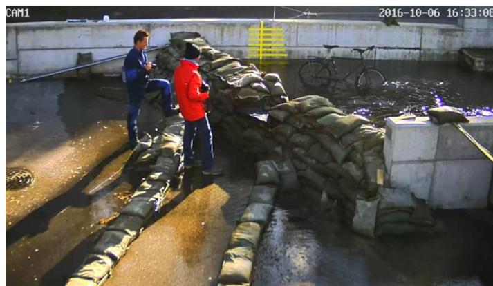
**Figure 2: View from camera CAM1 in which a bicycle is visible in the flood water behind the dam. Deep learning could make it possible to automatically estimate the water level from such an image. An ultrasonic sensor above the water and a pressure sensor in manhole m1 provide water level data.**
