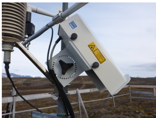
Figure C4. Laser snow depth sensor attached to the climate station, Bayelva, Aug. 2013–present, UTM: 33 N 432100 8762992.
