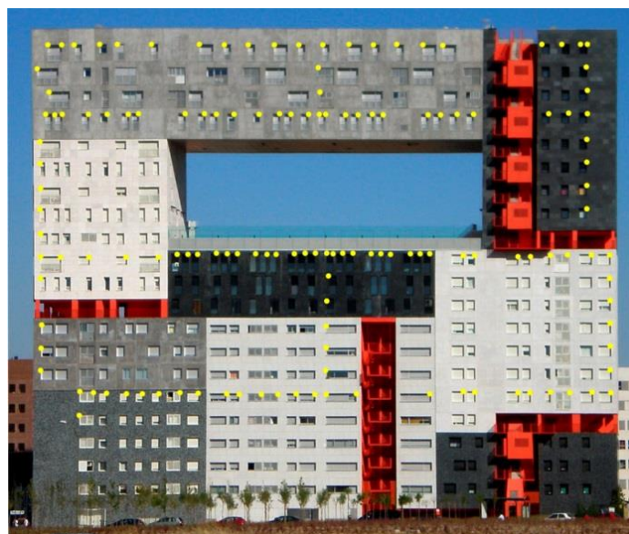
Figure 5. View of the facade of the building Mirador used for the calibration of non-metric camera used in photographic shots of Johnsons glacier front. Yellow, the measured points by using a total station.
