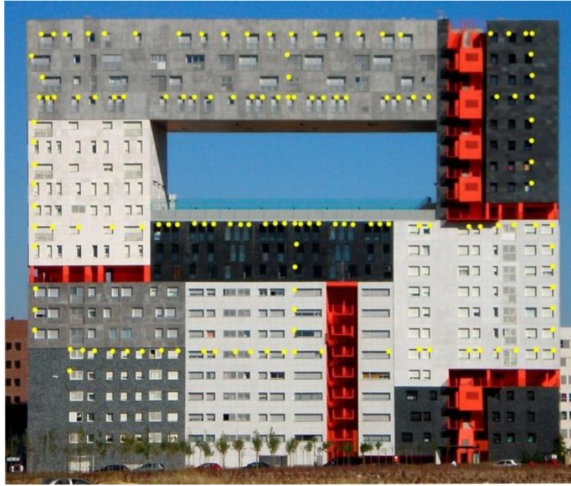
Figure 4. View of the facade of the building Mirador used for the calibration of non-metric camera used in photographic shots of Johnsons glacier front. Yellow, the measured points by using a total station.
