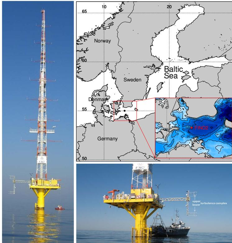
**Figure 1.** FINO2: position in the Baltic Sea (top, right), the measurement mast (left), and the platform with the boom and instrument installation at 6.8 and 13.8 m height above sea surface (bottom).
