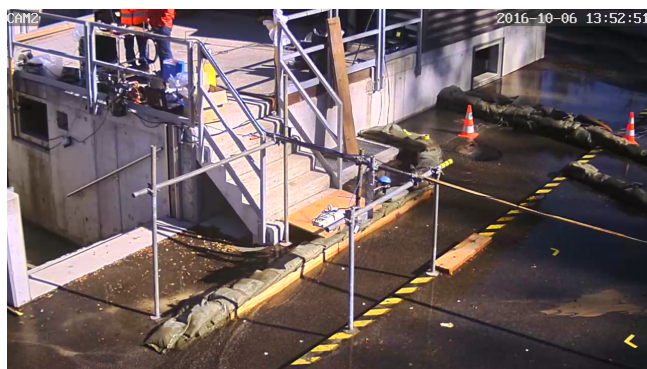
Figure 6. View from camera CAM2 in which channel c3 is visible, as well as the scaffolding holding two radar-based flow measurement systems. The same channel is also visible from camera CAM3.
