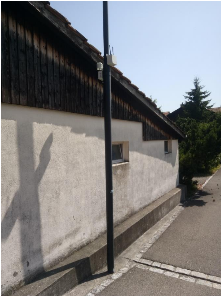
Figure S28. LoRa-Mesh repeater node (upper box) self-sufficient with the Solar Panel
