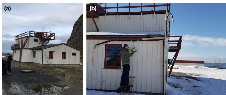
Figure A1. (a) Site Coast seen from SW direction with Adhauet mountain to the right. The Parsivel 2 disdrometer, Micro rain radar, and aerosol inlet are visible on the top of the building. (b) Heated inlet for water vapour isotope sampling at site Coast looking W towards the Norwegian Sea.
