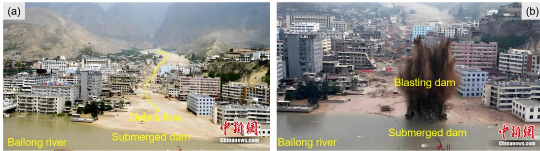
**Figure 1.** Post-disaster images of the Zhouqu debris flow. (a) The debris flow rushed into the Bailong River, forming a submerged dam; (b) blasting operations on the debris flow barrier dam to accelerate discharge. The images were obtained from China News Service (<https://www.chinanews.com.cn/>, last access: 15 February 2025).
