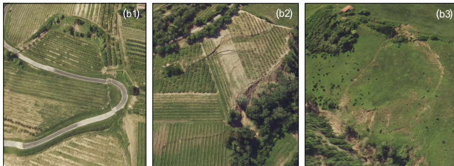
Figure 6. Representative images of the two distinct types of rock-block slides caused by the May 2023 event.
