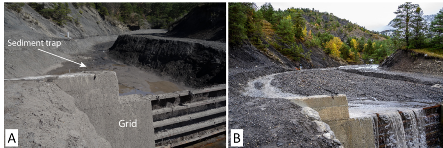
Figure 10. Sediment trap at the Laval station. (a) Trap is empty, and (b) trap is full. Photo a from Coline Ariagno. Photo b from Hubert Raguet).
