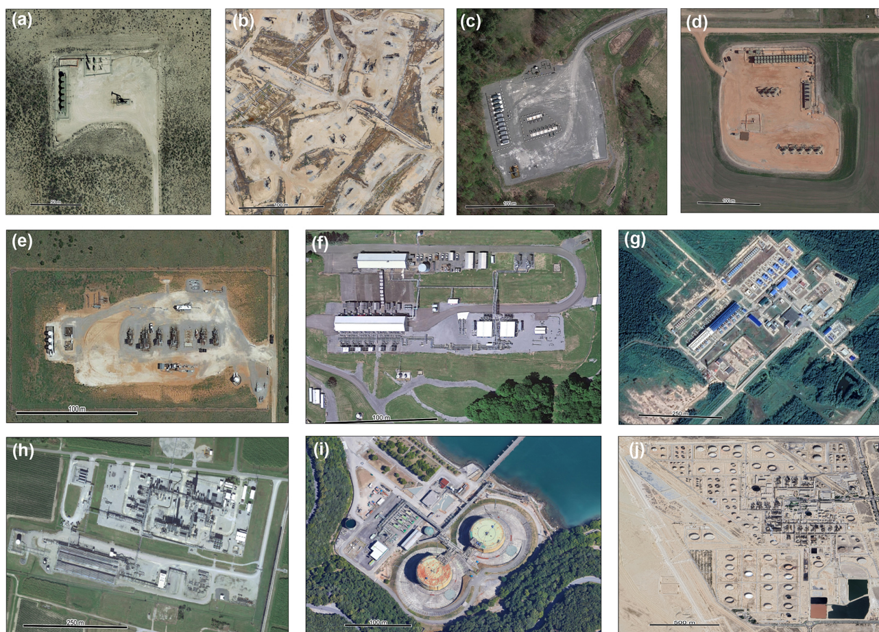
Figure 1. Examples of major oil and gas facility types as seen in high-resolution satellite imagery (Google basemap imagery, © Google Earth). (a) An oil well pad with one pump jack and storage tanks in the Permian Basin, United States. (b) A cluster of oil pump jacks in the Kern River Oil Field in California, United States. (c) A dry natural gas production well pad, with 11 horizontally drilled wells, in the Marcellus Shale play (northeastern Pennsylvania, United States). (d) A mixed oil and gas production well pad in the Bakken Shale play (North Dakota, United States), with eight horizontally drilled wells. (e) A natural gas gathering compressor station in the Anadarko Basin (Oklahoma, United States). (f) A natural gas transmission compressor station in Pennsylvania (United States). (g) A natural gas transmission compressor station in the West Siberian region (Russian Federation). (h) A natural gas processing plant in Louisiana (United States). (i) An LNG regasification facility in La Spezia, Italy. (j) A crude oil refinery in Mesaieed, Qatar.
